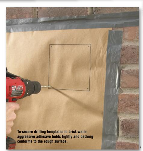
Among the many proven 3M industrial tapes, this is the duct tape engineered as a "power" tool for demands throughout many work sites. Power is in the high 30 lbs./in tensile strength and the hefty 10.7 mil tape thickness.
