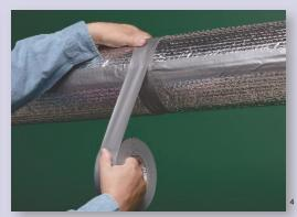
Polyethylene coated cloth with rubber resin adhesive conforms and adheres to seal around insulation and duct work.
