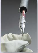
Bundled electrical wires are easier to pull through conduit. And for less bulk in the conduit, 3M<sup>™</sup> Duct Tape 3900 Tape provides the lowest profile of all 3M
